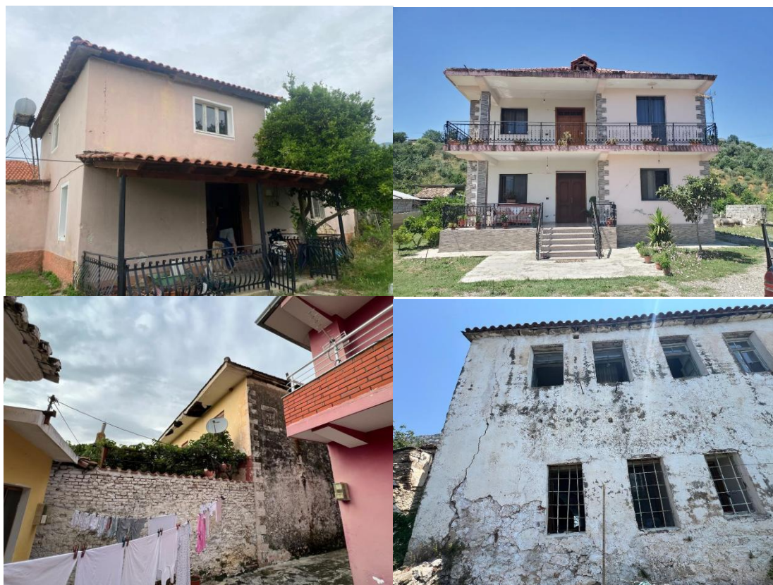
Figure 1. Building façade view brick URM building 1,2 (up left and up right) and stone URM building 3,4 (bottom left and bottom right)
