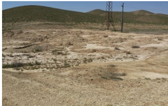
Figure 9. Areas where reclamation systems have collapsed
